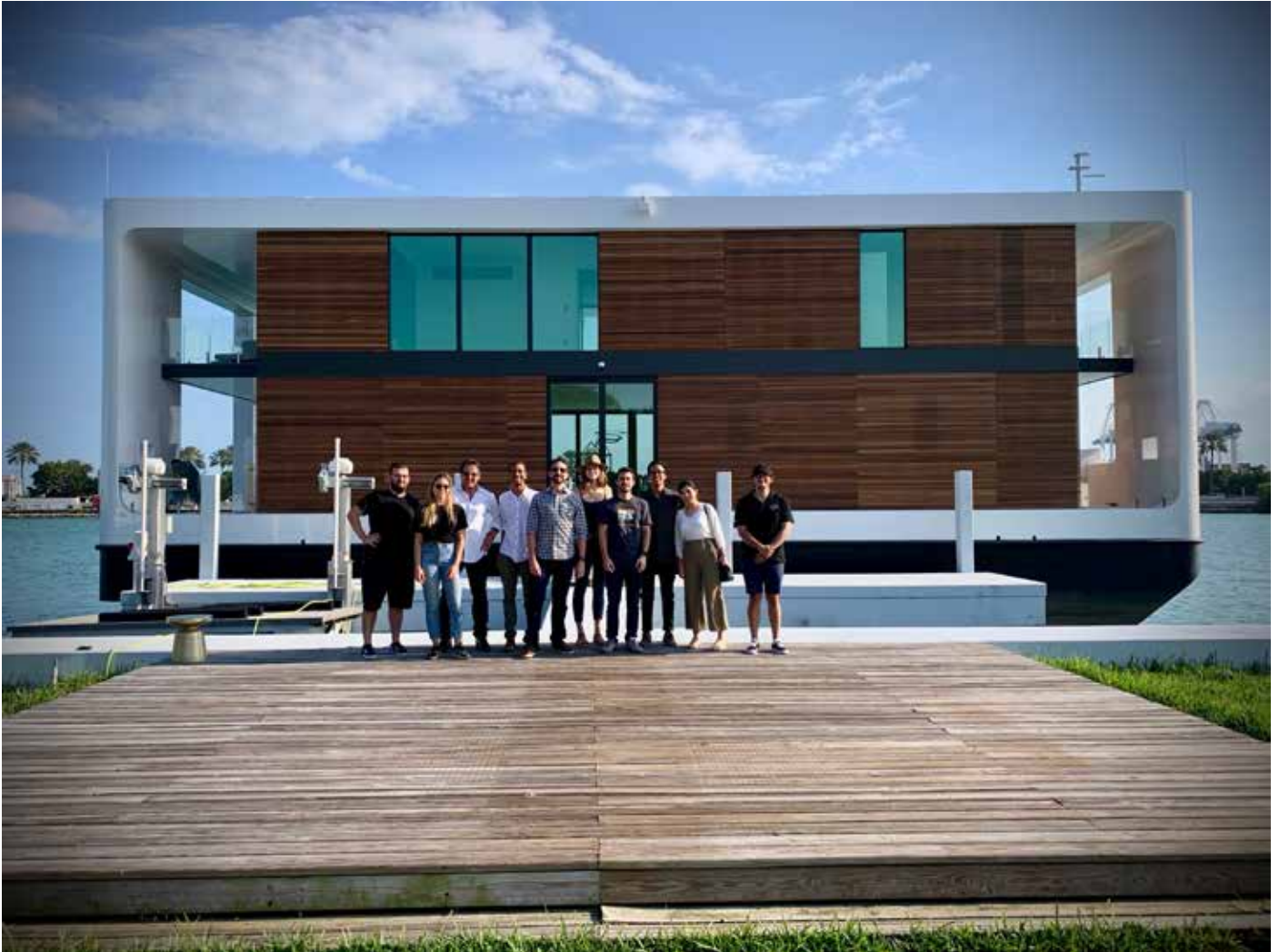
CRUNCH researchers visit the arkup hybrid during its visit to Star Island in the City of Miami Beach. The arkup hybrid is a sustainable floating residence that can adapt to sea level rise and can withstand hurricane force winds and storm surge. https://arkup.com/
