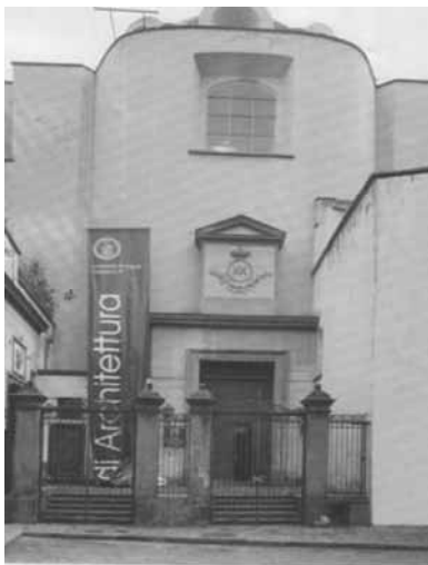
Fig. 1. The church of San Demetrio e Bonifacio, now Aula Magna of the Naples' Architecture Department
