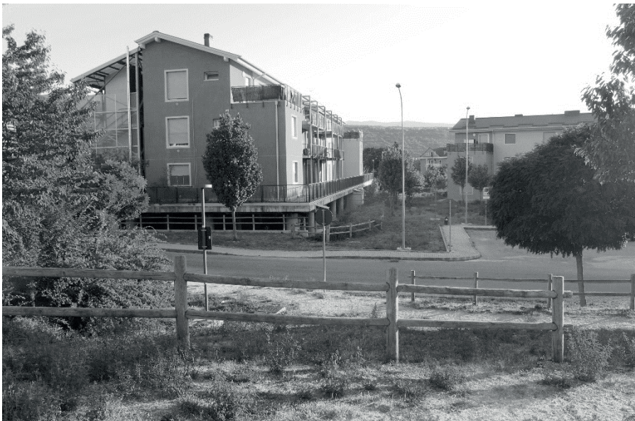
Fig. 1 - The new town of "Sant'Antonio" in L'Aquila, 2020
